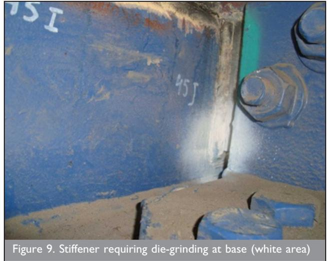
Figure 9. Stiffener requiring die-grinding at base (white area)
