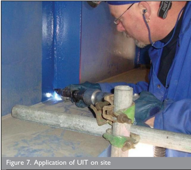
Figure 7. Application of UIT on site
